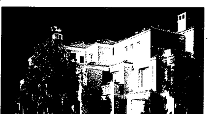
San Paulo Apartments, Irvine, CA 25 Units/Acre
