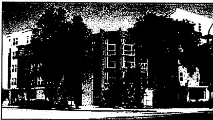
Coggins Square Pleasant Hill, Walnut Creek, CA 42 Units/Acre
